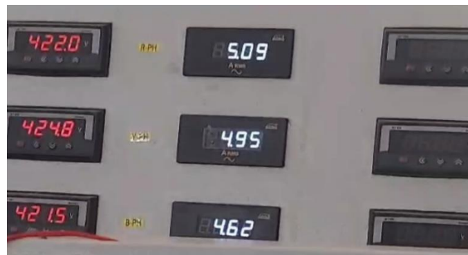
Figure.5. Before turning on the capacitor bank our current is 5.2A
