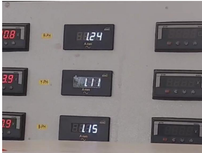
Figure.7. After turning on the capacitor bank our current is 1.3A
