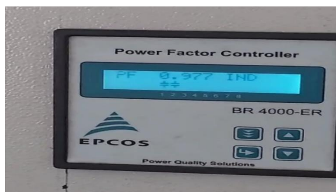
Figure.6. After turning on the capacitor bank our Power factor is 0.977
