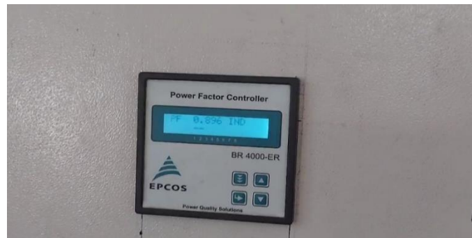
Figure.4. Before turning on the capacitor bank our power factor is 0.896
